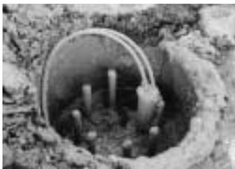
When the piling is finished, the area enclosed by it will be dug out. If all goes according to plan (and the weather has been surprisingly kind so far) work on the basement floor will begin in May.
