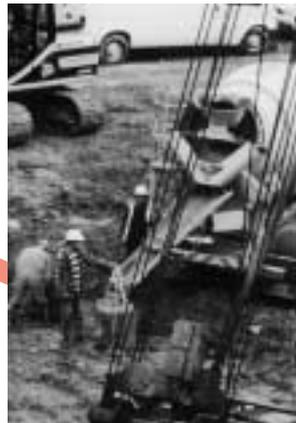
◀ This is the concrete being poured in the tube that holds the cage that holds the pipes
