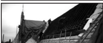
The now-regular roofing work continues — here above Hall.
