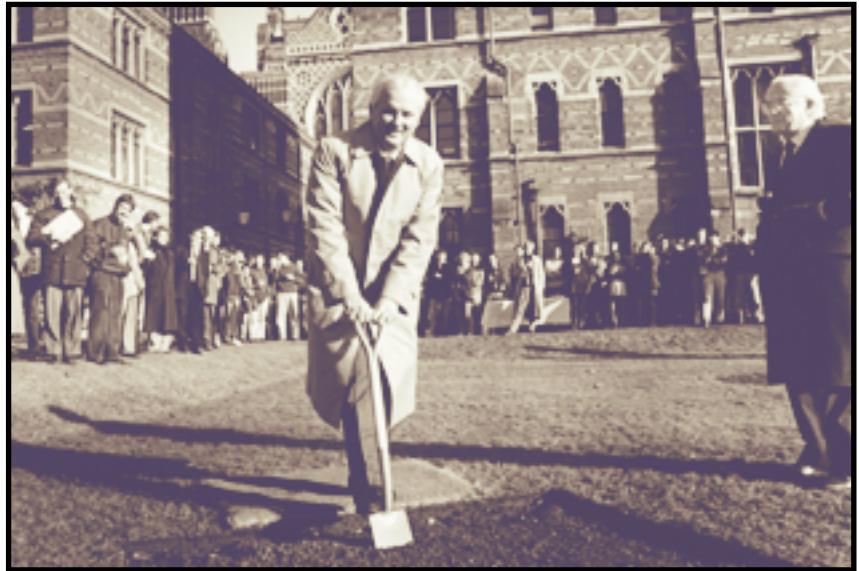
December: The Warden looks on as Lodwick Cook, Chairman and Chief Executive of Arco, turns the sod at a ceremony marking the start of construction on the new Arco Building
